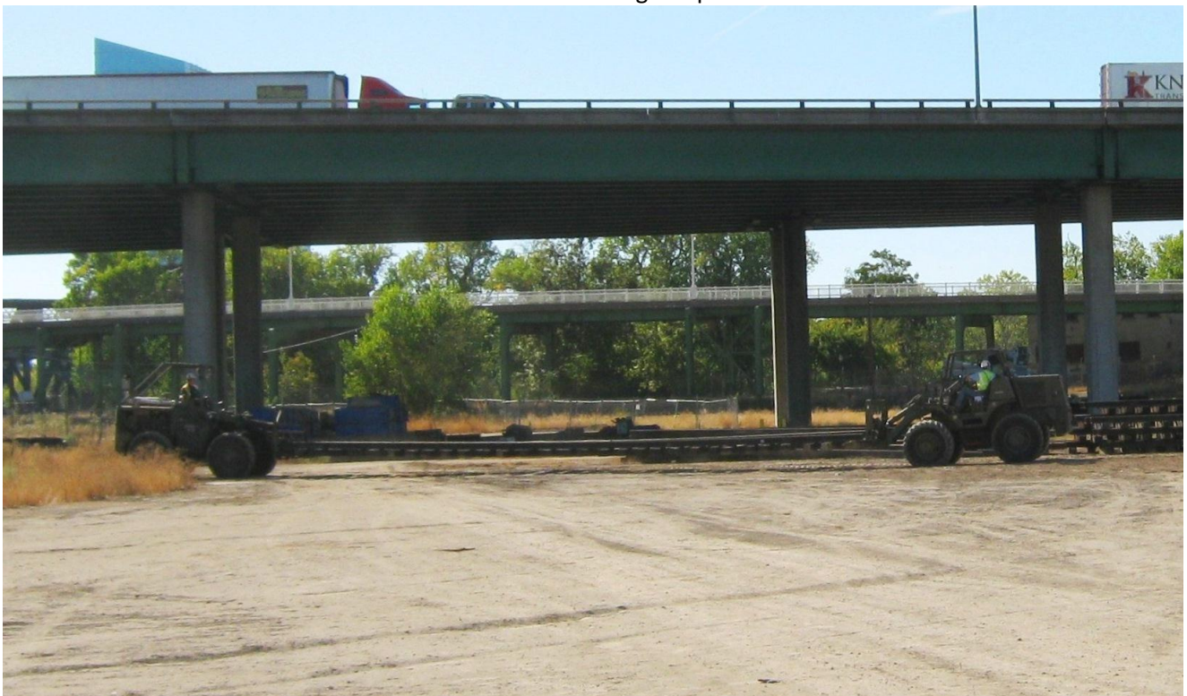
For perspective, here's an historic photo of both Green Machines moving a section of panel track from October, 2012.
