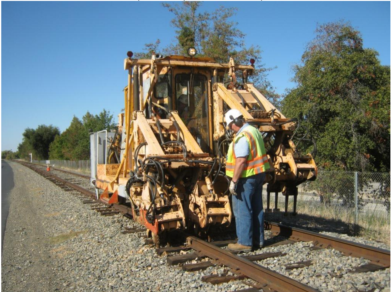
Chris guides the tamper's actions in raising the west rail
