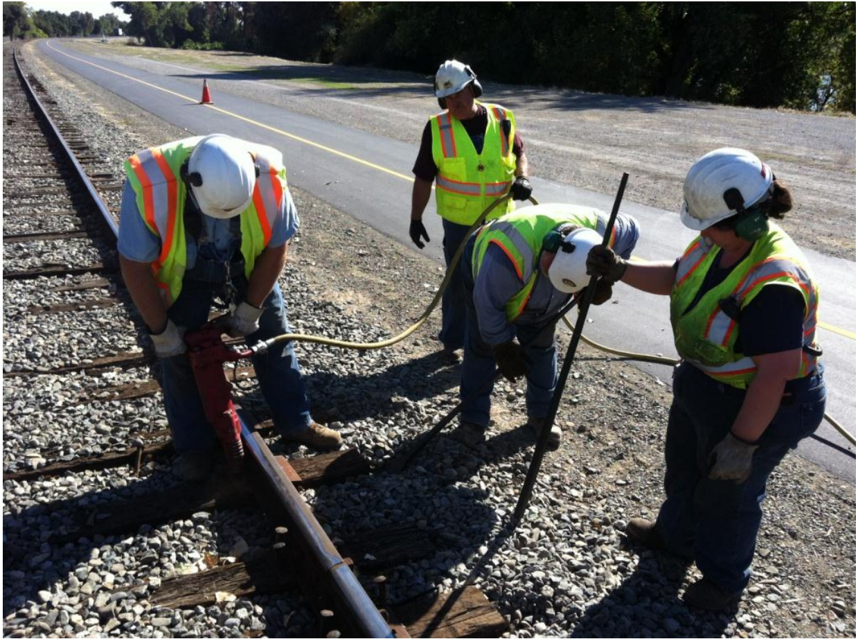
Chris uses the pneumatic spiker while Frank "nips" the track
